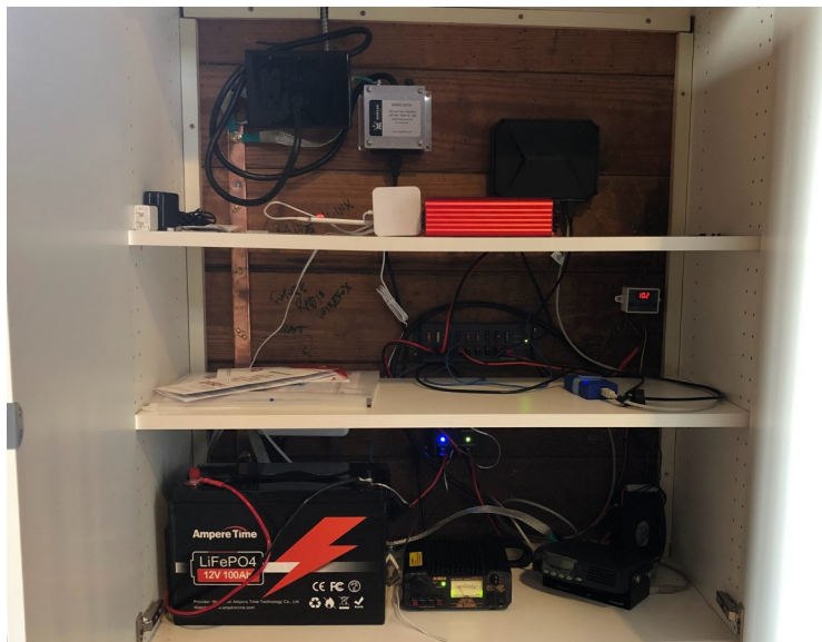
The completed station with room for storage and expansion
