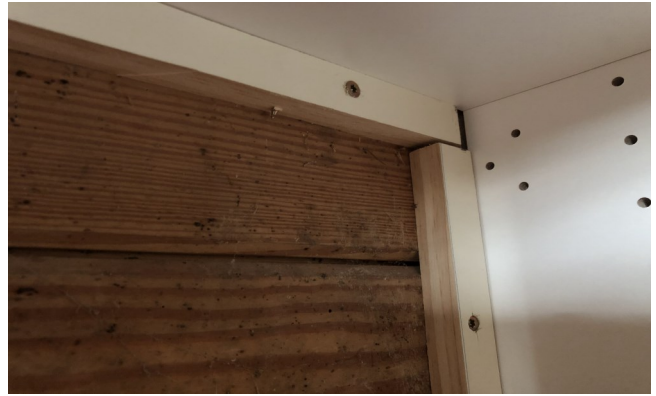
Detail of attachment to barn wall.
