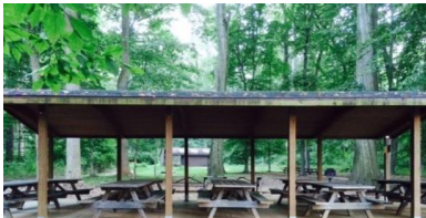
Pavilion #14 at Ridley Creek State Park waiting to be occupied
